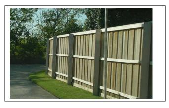
The materials and color for any fence construction must be approved by the ACC. Boardon-board construction in natural cedar is an excellent example of a fence design.
